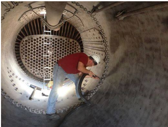
Will Sadler, 611 mechanical volunteer, works inside the boiler, vacuuming debris left from the bead blasting.
