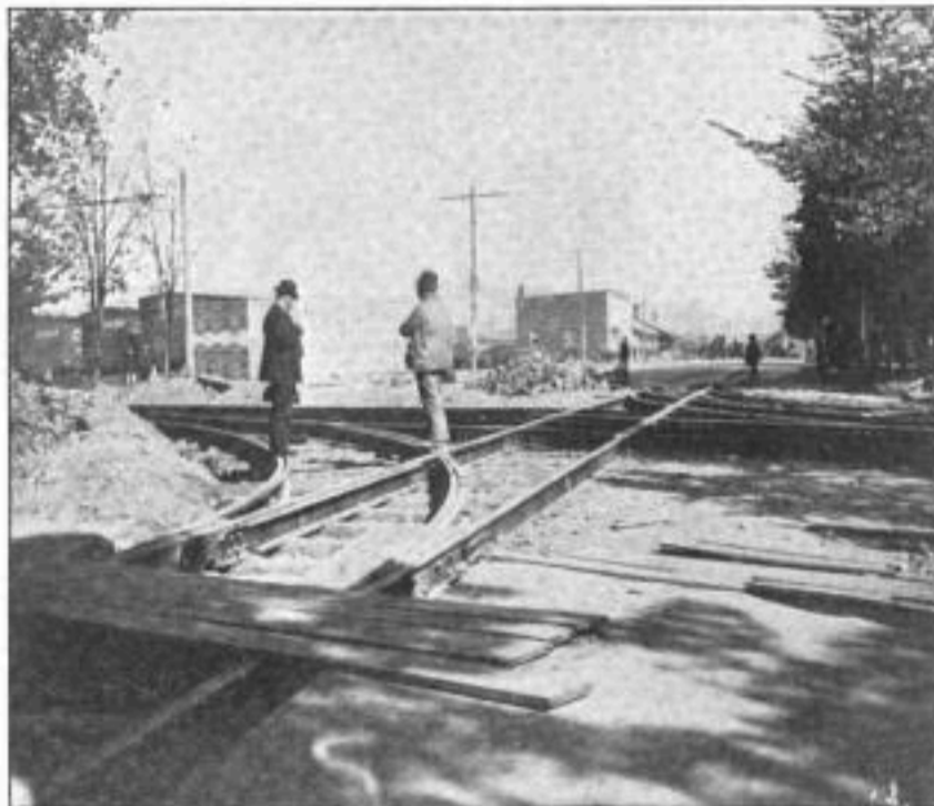
FIG. 6.—GIRDER RAIL CONSTRUCTION.
