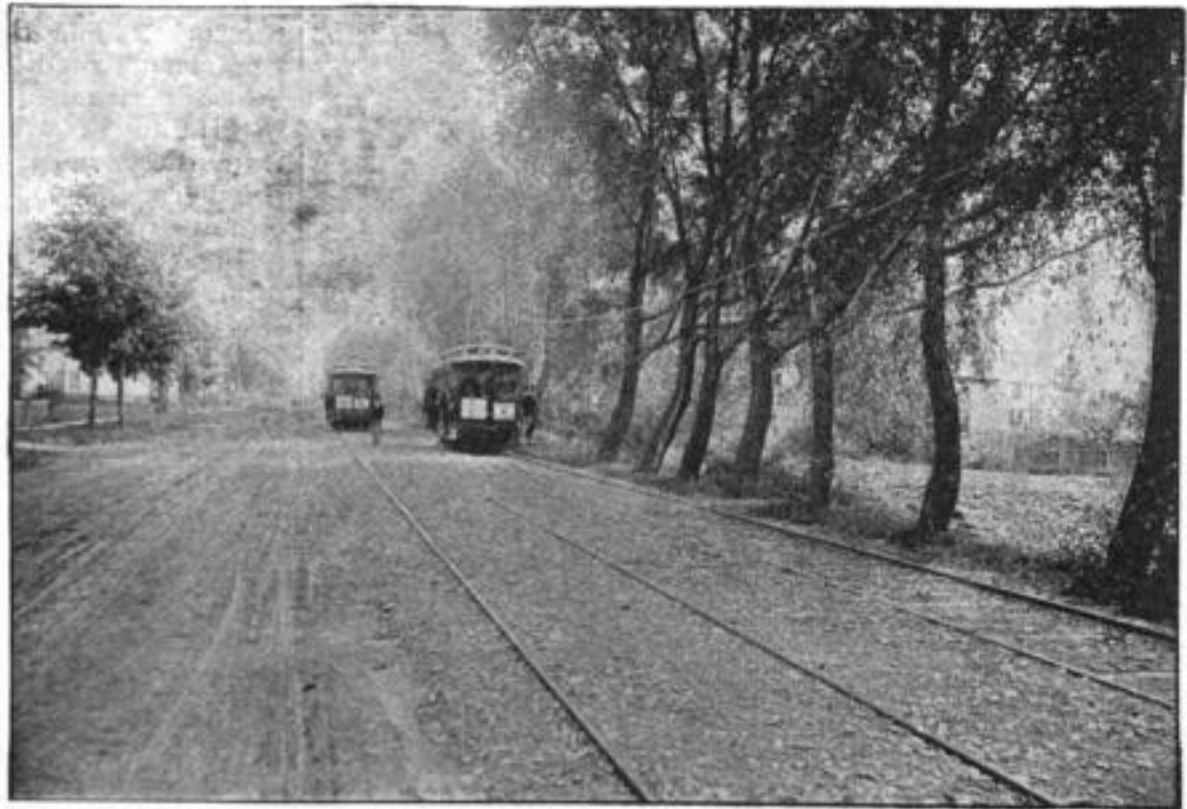
FIG. 4.—T RAIL CONSTRUCTION—PARK AVENUE
