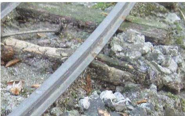
At Melaleuca the rotting sleepers are a serious defect, even if on a siding.
