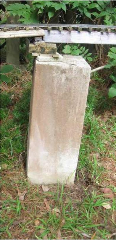
The long girder bridge leading to Ti-tree has piers leaning in a dangerous manner. This picture shows the main pier and the very temporary measures taken to try to counteract the sinking pier.
