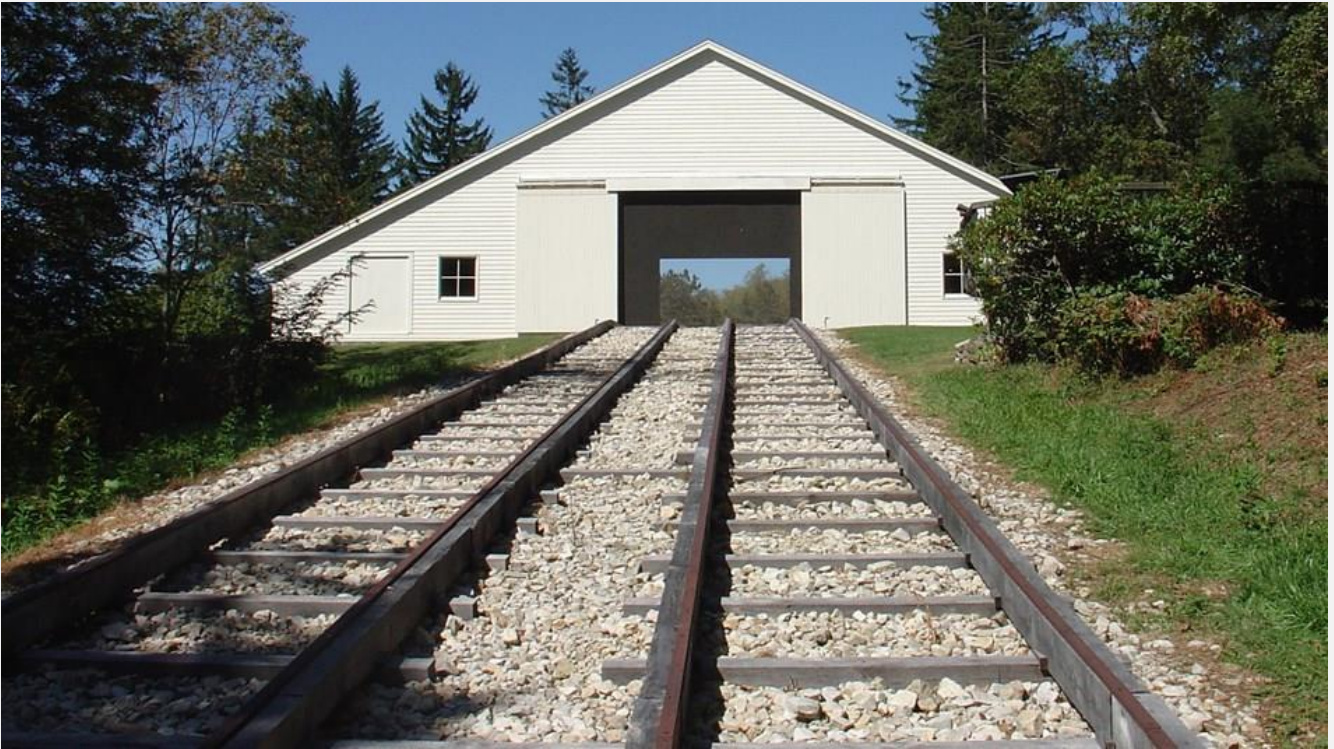
The National Park Service has reconstructed segments of the railroad. Note that the “rail” here is wood beams capped by iron straps to reduce wear and friction.
