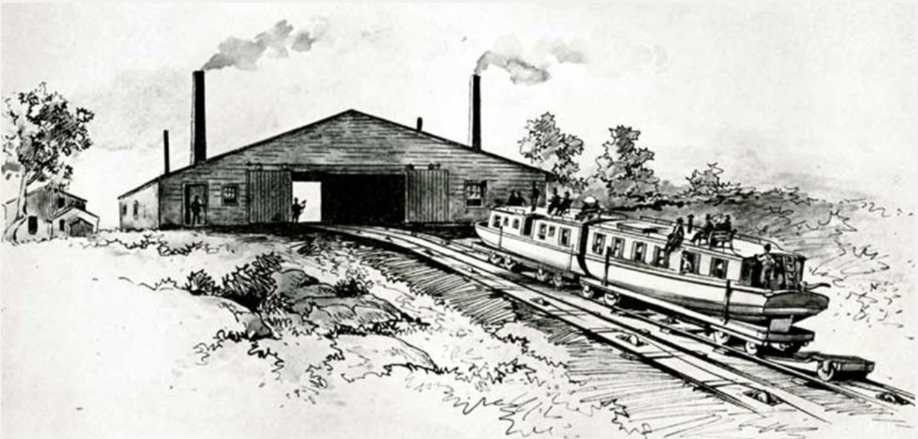
A drawing of boats being pulled upgrade. I'm not sure I would want to sit on the roof if a cable broke.
