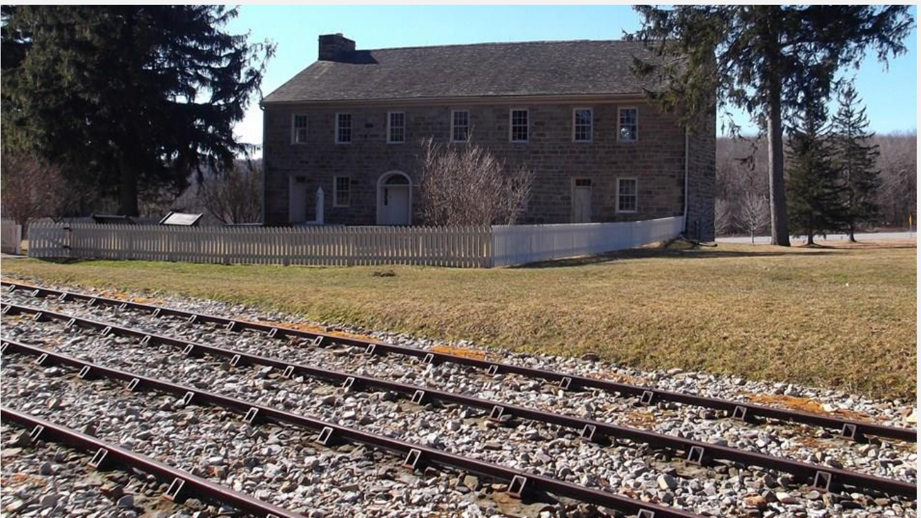
Another segment of the railroad has been preserved at the Summit. The structure in the background is the Lemon House where canal patrons could receive refreshments. Note that iron rail has replaced the wood beams and is chaired not on wood ties but on stone blocks sunk into the earth.
