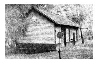
First it was necessary to make drawings. Because there is no direct frontal view of the depot, I made measurements of the windows and doors from both photos, then averaged the dimensions to compensate for differences due to perspective. Originally I had no photo of the rear of the building so I didn't know if there were windows there. Since I had only four window castings (Tichy #8030), I opted to add windows only to the front and east sides.
