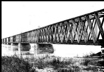
Truss Bridges: The Howe Truss
