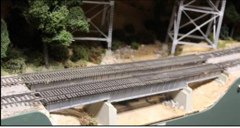
Three-span Deck Plate Girder
