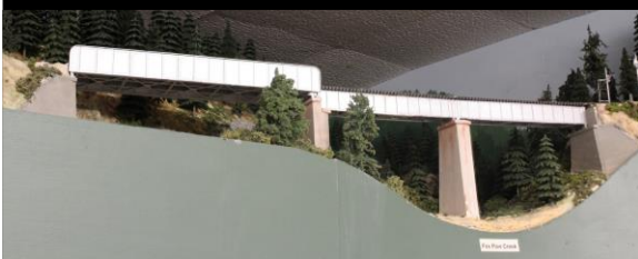
Combination Through and Deck Girders
