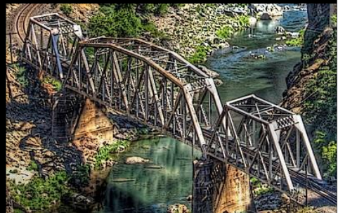
Warren Truss, Pulga, CA
