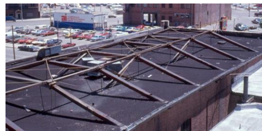
Exterior roof trusses
