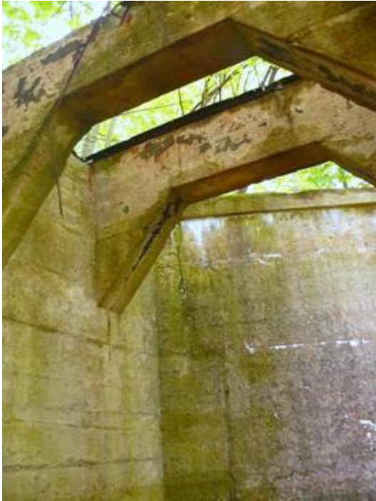
Coal bunkers from rail siding access overhead.
