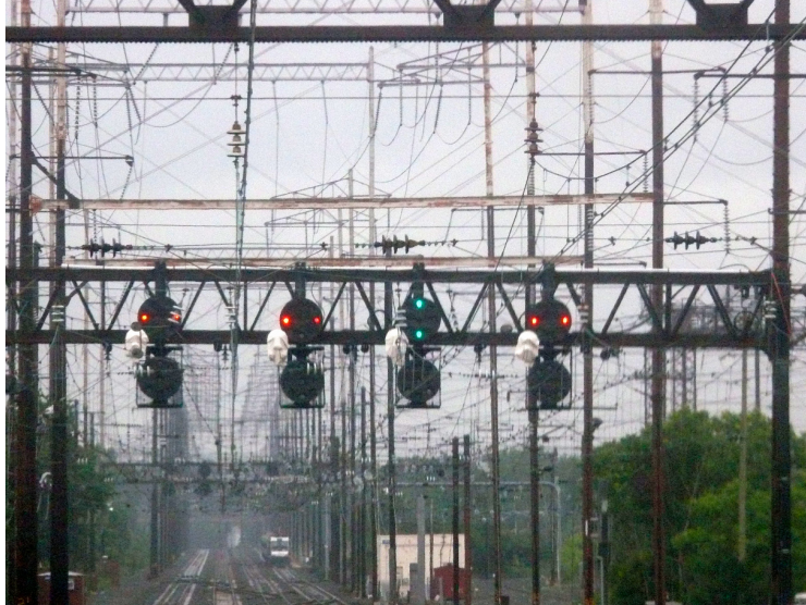
Illustrates position-light signals on the corridor utilizing two bulbs per aspect, red, green, amber...similar to that used in prior years on the Norfolk & Western RR.
