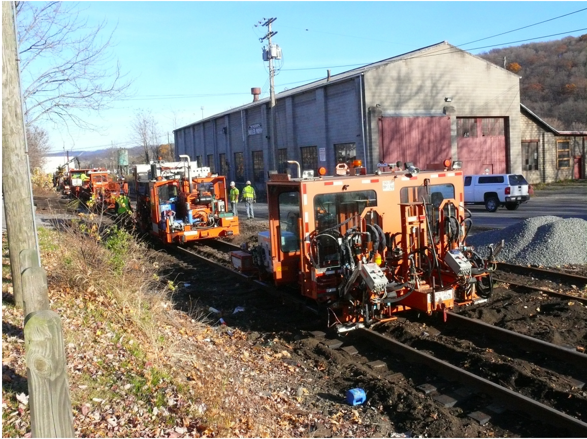
Norfolk Southern track crews re-build the main track entering Hollidaysburg Yard.
