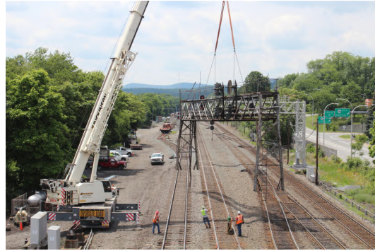
Picture 4: Slope Westbound Signal Bridge being lifted from its foundation and moved trackside. 1:21 PM.
