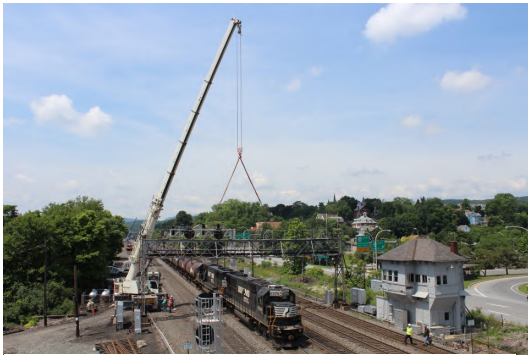
Pictures 2: ALTO Eastbound Signal Bridge being lifted from its foundation. 1:06 PM.
