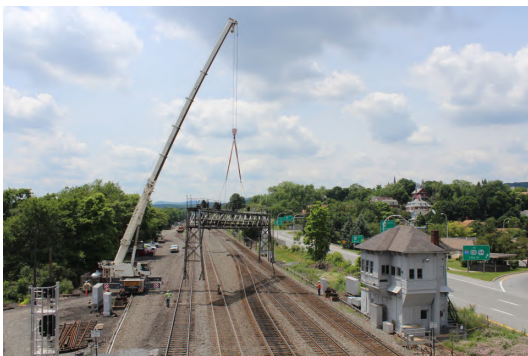
Picture 3: Another view of ALTO Eastbound Signal Bridge being Lifted.
