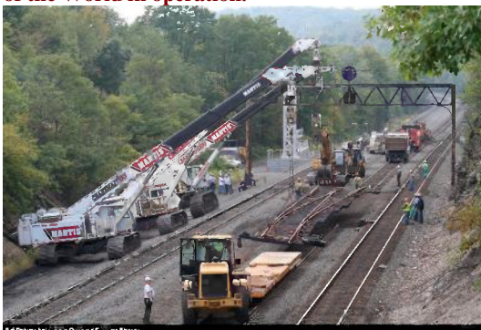
Replacing SLOPE interlocking 9-23-2011. Photo by Jamey Rickens; used with permission.
