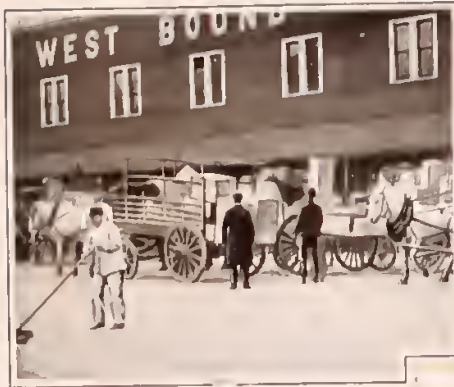
Waiting at a Freight Station — Manhattan.
