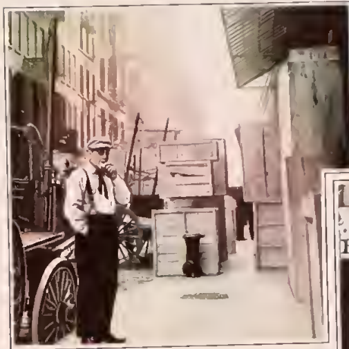
Truckman waiting for the elevator to bring down part of a shipment from a Loft in Manhattan.
