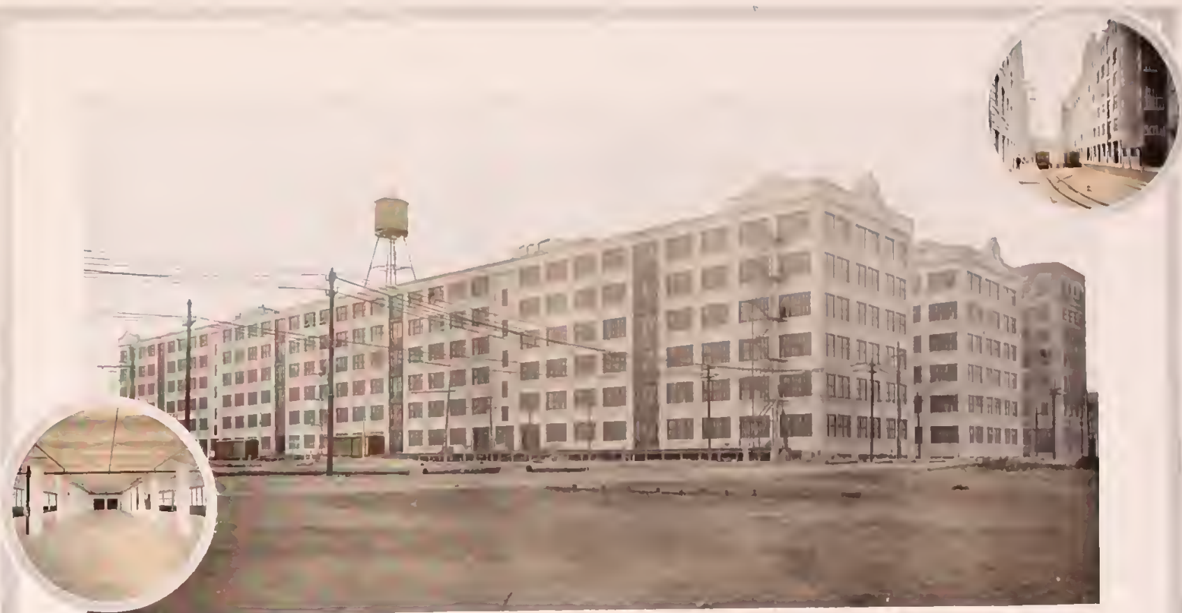
VIEW OF FOUR OF THE ENORMOUS MODEL LOFT BUILDINGS
