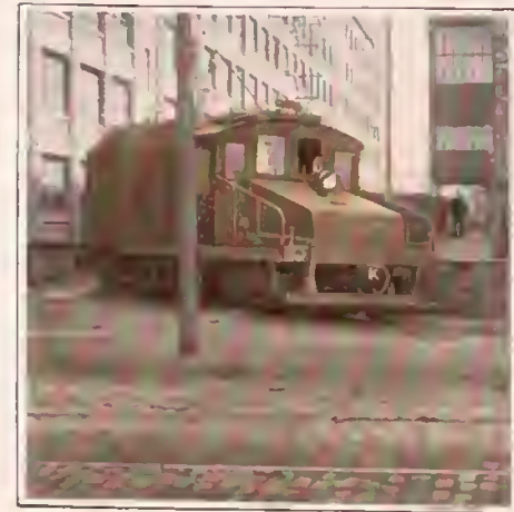
Bush Terminal electric switching engine starts the shipment on its way without delay.
