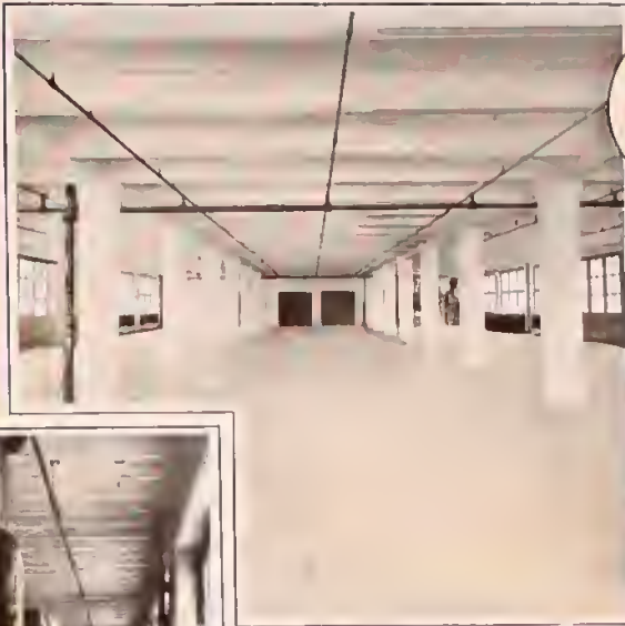
Typical space in our Model Loft Buildings, showing unobstructed floors and perfect light
