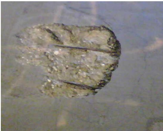
*Pothole in Stamford garage showing exposed rebar.*
