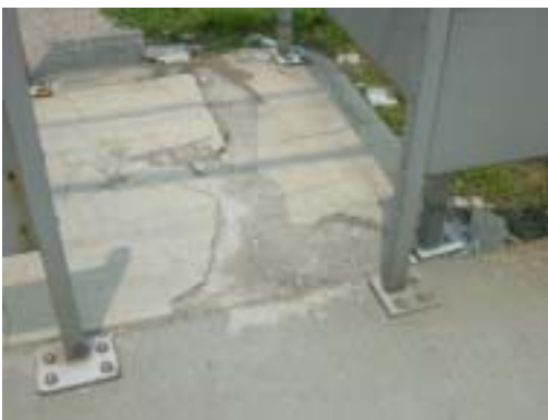
Cracked concrete.
