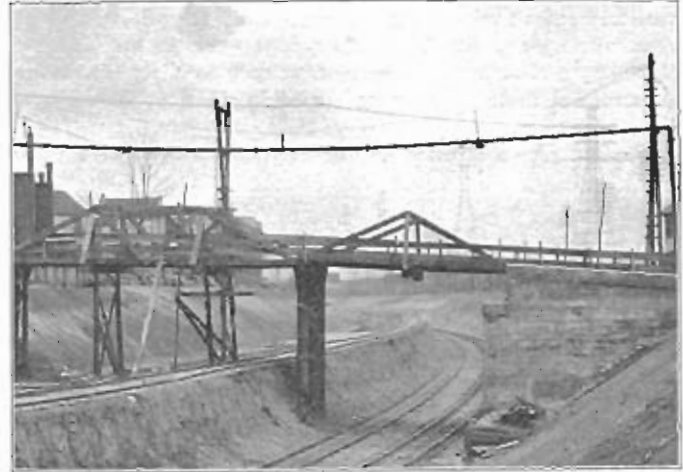
Looking East at Dunn Street After the Third Shovel Cut.
