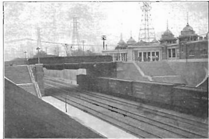
Dufferin Street Overhead Bridge at Entrance to Exhibition Grounds.
