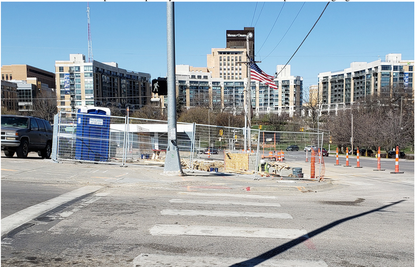
4/10/2020-Sidewalk view looking west across Park Ave. No pedestrian path around construction site, and no signage.
