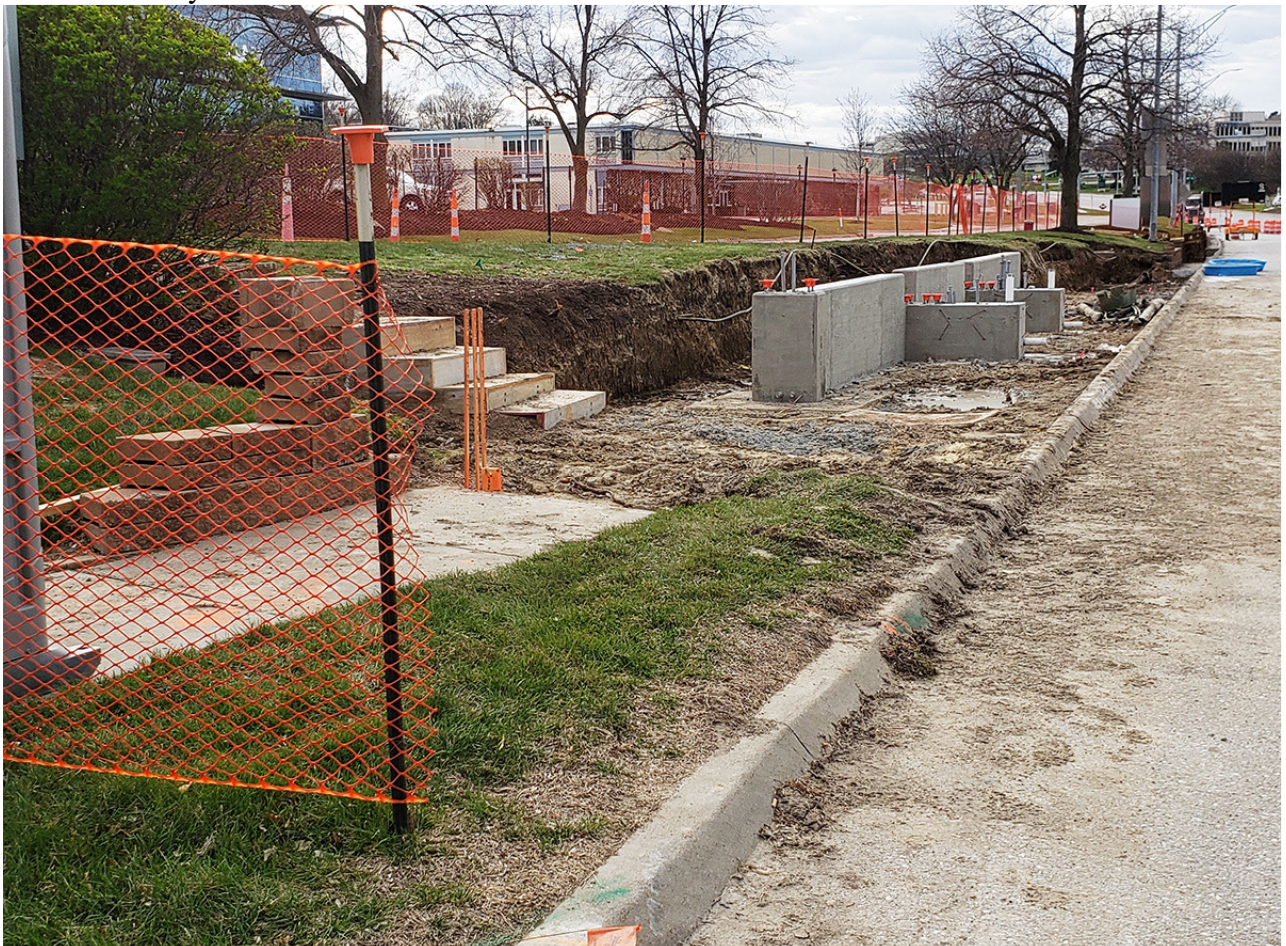
4/20/2020-View looking west from 84 th St. towards the station site. Note there is an existing sidewalk on the left, and it may have led to a O-Metro bus stop at this location. A new stairway leading from the ORBT station to the sidewalk and frontage road is being built as part of the project. Wheelchair passengers will be able to use the sidewalk leading to 84 th St.
