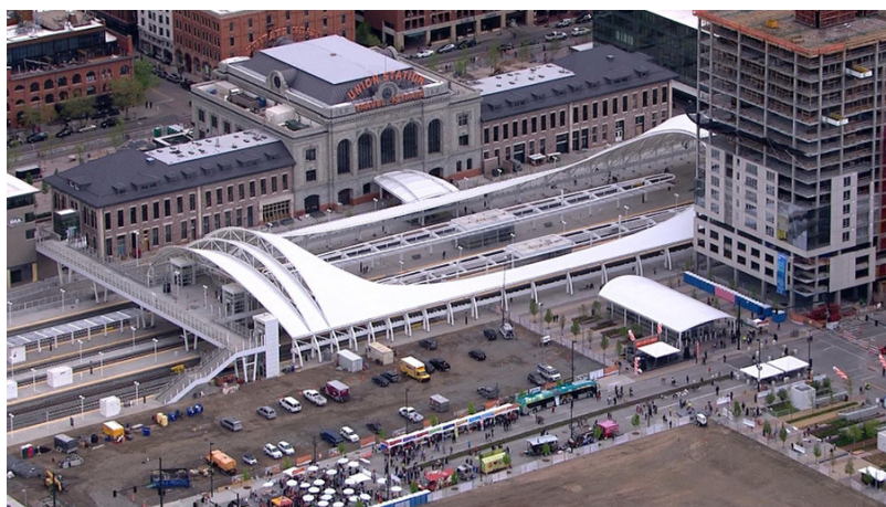
Denver Union Station Transportation Center (RTD Photo)
