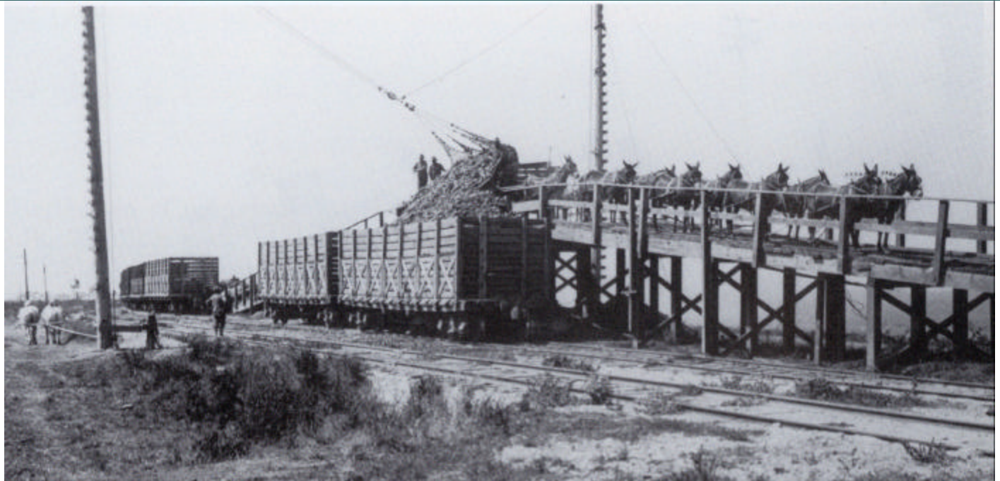
Figure 2. Narrow gauge beet racks in San Luis Obispo. The racks with side opening doors were mounted on flatcars during beet season. Photo from the collection of Thomas Petersen.
