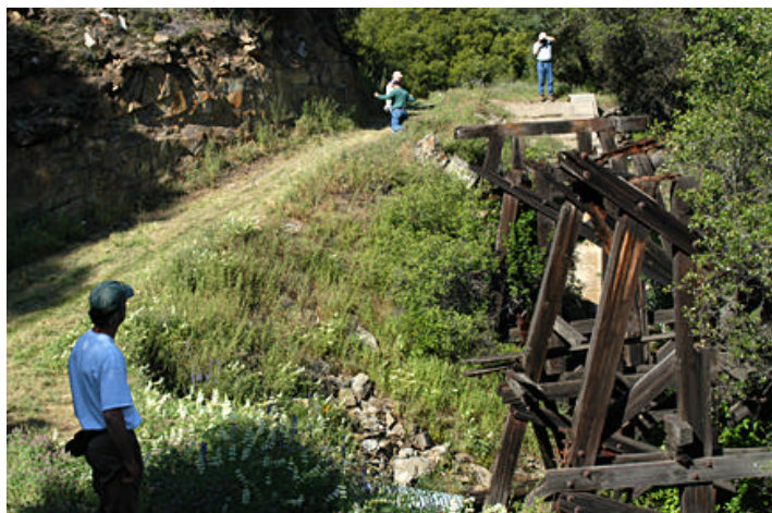
Checking out the trestle near Briceburg. 17 May 2003 photo by Jack Burgess.
