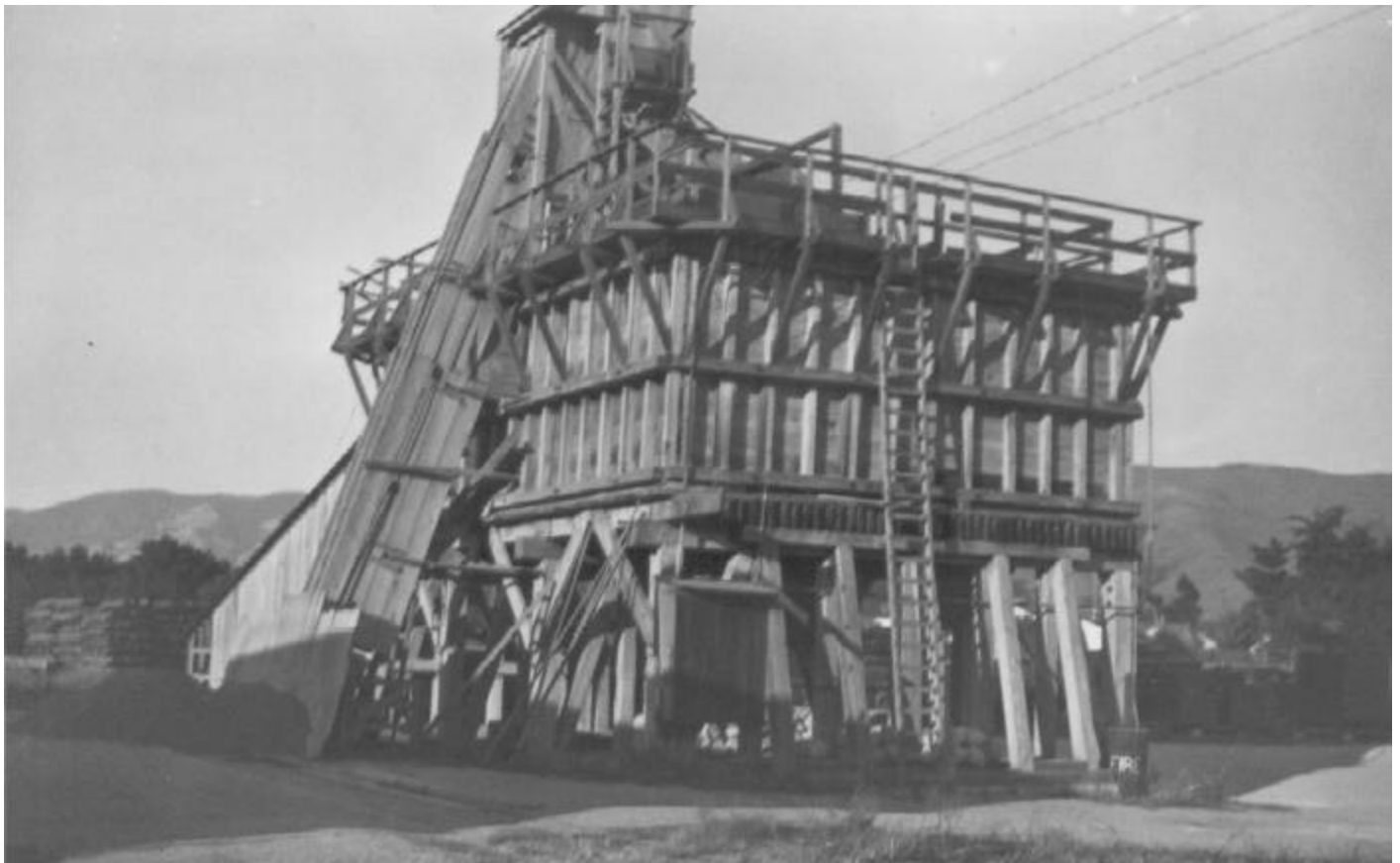
Figure 4: The gravel bunker located at the facilities of the Pacific Coast Coal Company in San Luis Obispo. The PCRY tracks are located in the foreground at the left. Credit: Kenneth E. Westcott as published on page 135 in The Pacific Coast Railway: Central California's Premier Narrow Gauge by Westcott and Johnson.
