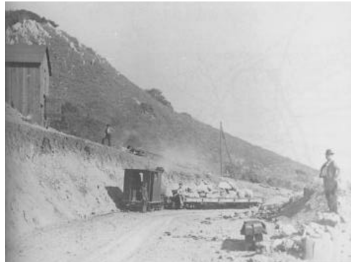
Figure 2: Bishop Peak Quarry Operations. This view taken prior to 1908 when the quarry shut down shows a narrow gauge flatcar about to be lowered down the incline toward Foothill Boulevard and then transferred out to Avila. The quarry offices and cable hoist house are at the left. Credit: San Luis Obispo County Historical Society as published on page 105 in The Pacific Coast Railway: Central California’s Premier Narrow Gauge by Westcott and Johnson.
