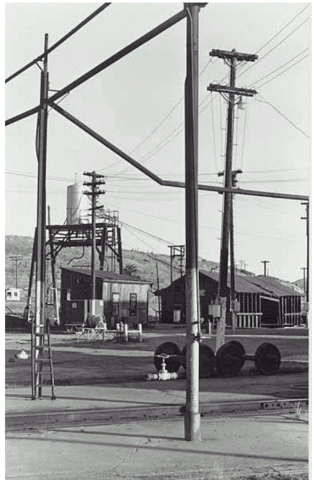
Figure 4: Sand house area from the southwest side. The photo also shows the related structures such as the sand tower, the battery plant and the numerous other poles, water hydrants and supports for the steam lines that were so characteristic of the SLO engine service area. Photo: Andrew Merriam, 1972
