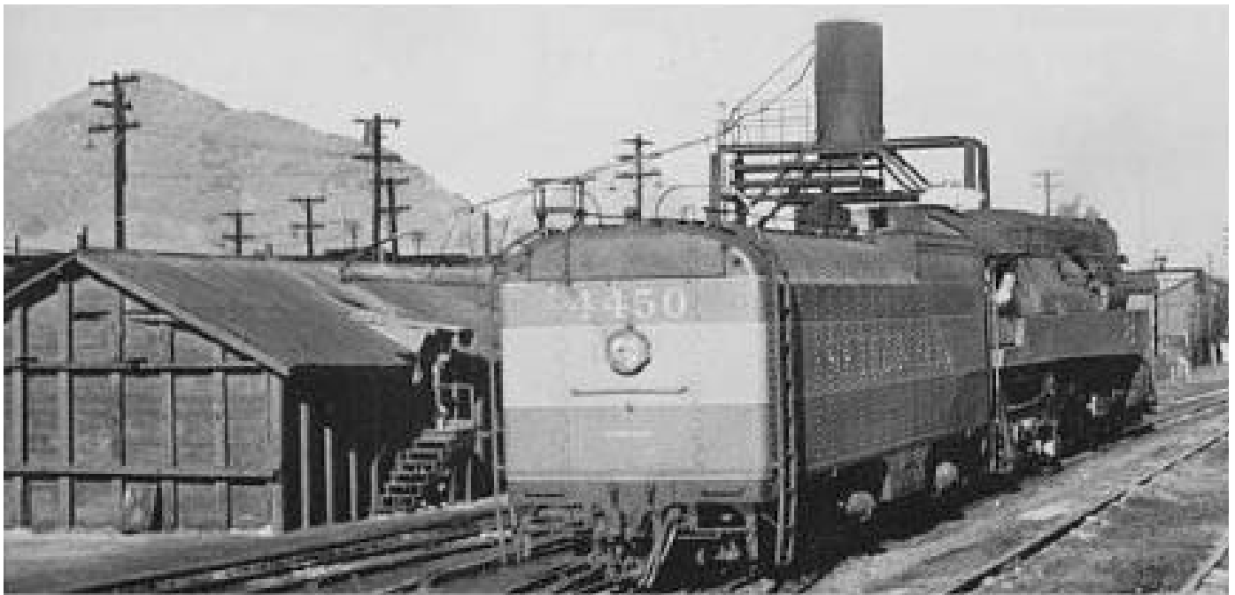
Figure 1: The sand house is to the right of daylight painted Northern 4450 (GS-4) which is ascending the ready track and heading toward the passenger depot in February 1954. The wood columns and horizontal girts which give the sand house its distinct character are clearly visible. Photo: With permission from Rod Crossley
