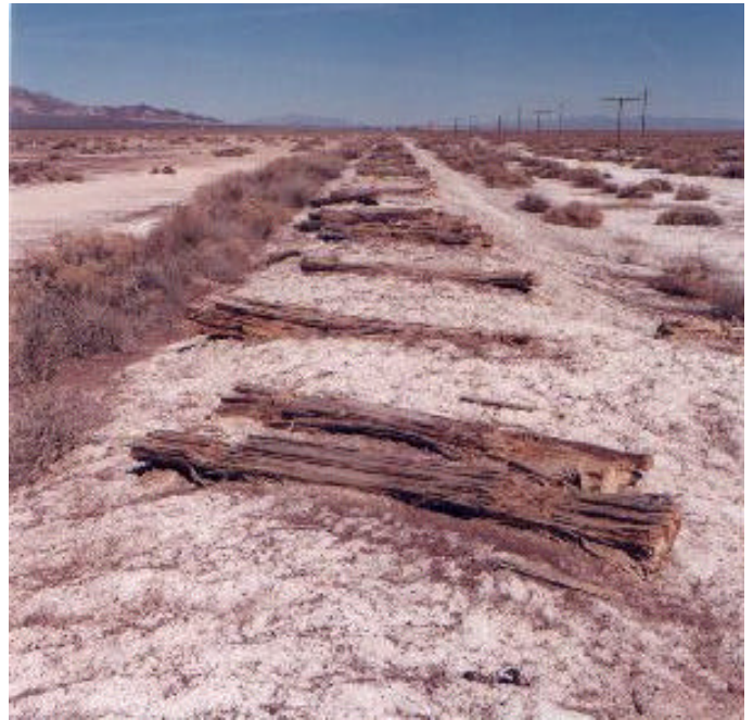
View along grade towards Death Valley Junction from same spot as at left. The abundance of ties is limited to this section. John Brabyn Photo.
