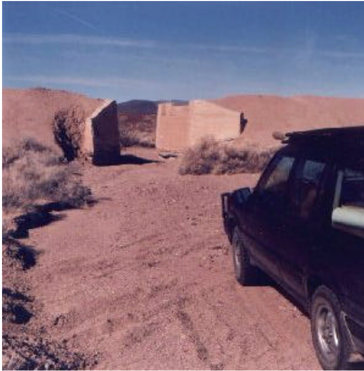
Approaching the old bridge abutments; T&T grade raised in background. John Brabyn Photo.
