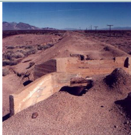
View near Eagle Mountain looking along grade towards Death Valley Junction. Bridge showing old wood and newer concrete abutments. John Brabyn Photo.
