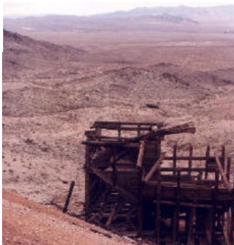
View from the Gunsight Mine towards Tecopa. Upper ore bin in foreground, lower bin in background, formerly connected by a dual car funicular. The Tecopa RR grade leaves the lower bin and skirts the hillside diagonally across the middle of the image. John Brabyn Photo.
