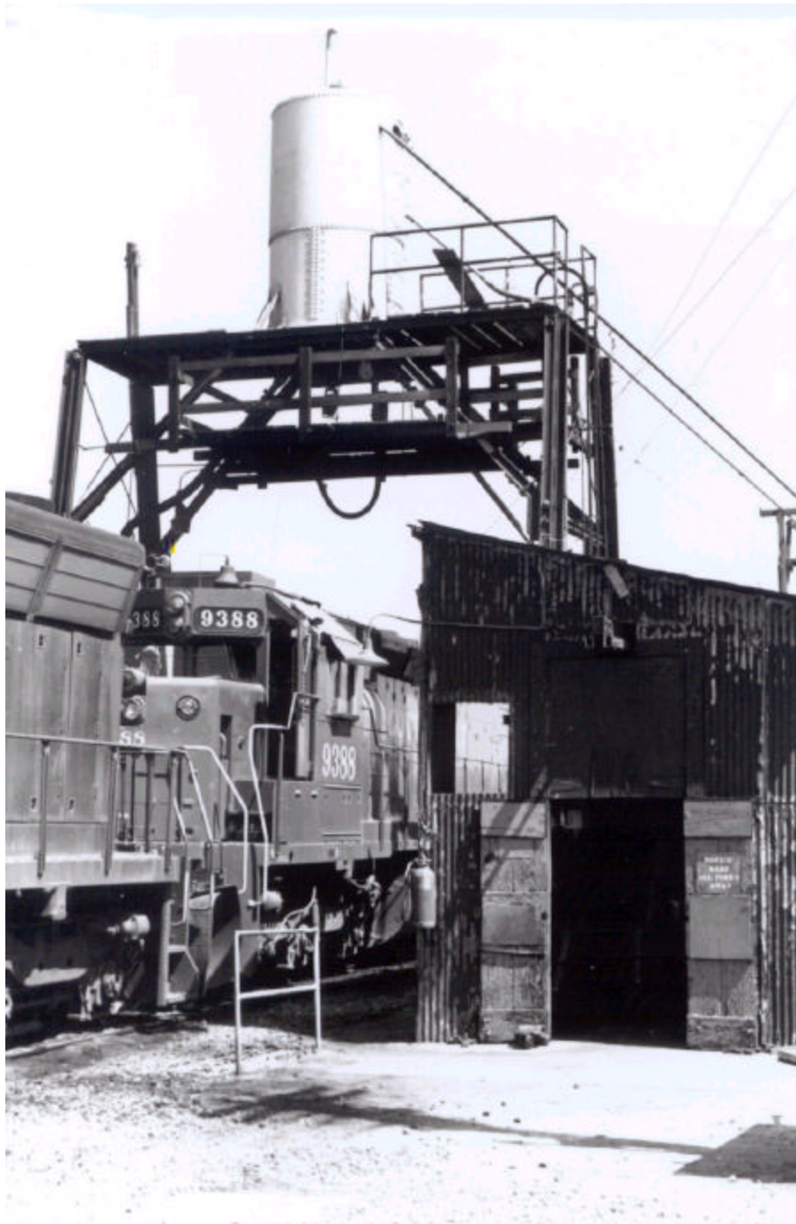
Figure 5: Detail Photo (1970) showing added details in the diesel era. The rail connections are visible from this angle as is the lower deck at the tank outlet. Credit: Andrew Merriam
