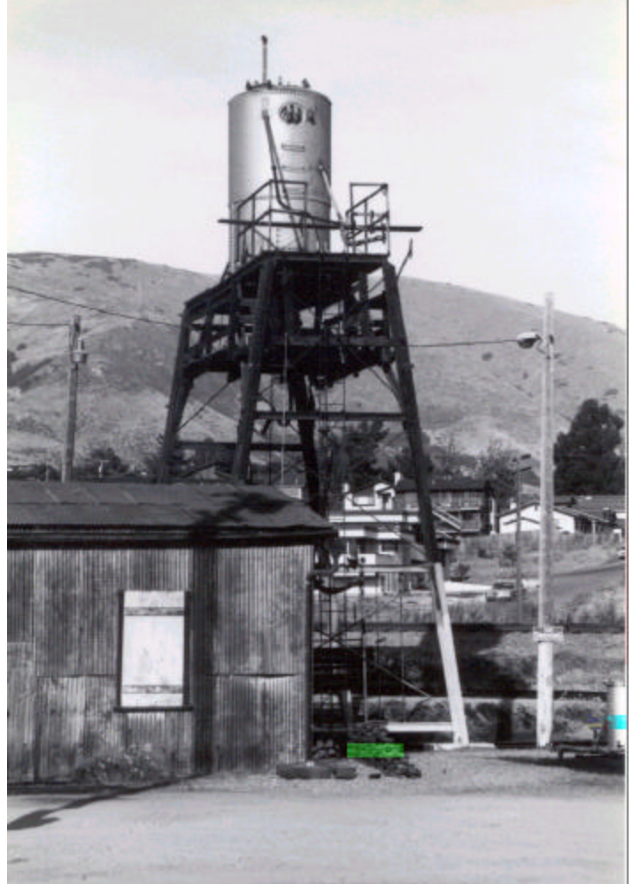
Figure 6: Side view of the sand tower after decommissioning. Note safety paint at the lower level. Credit: Andrew Merriam circa 1980s
