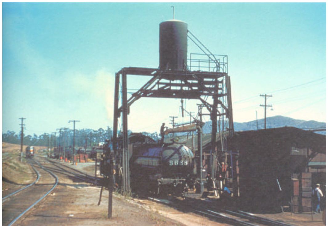
Figure 1: Photo of Sand Tower area circa 1954 with steam engine 3688 and F-4 pulling up to the water plug between the sand house and the sand tower. Credit: Alden Armstrong.
